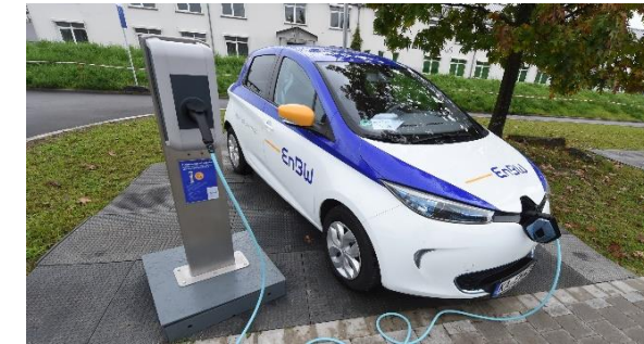
E-mobility charging infrastructure
